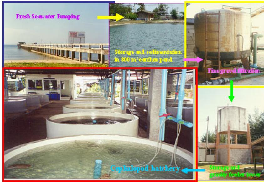
**Figure 1.** Seawater supply system in Rayong facility for cephalopod seed production and research activity.
